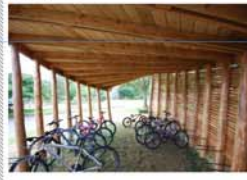
The hyperbolic paraboloid shape was generated by the desire to create a self shading structure to protect bikes and students from the sun and driving rain
