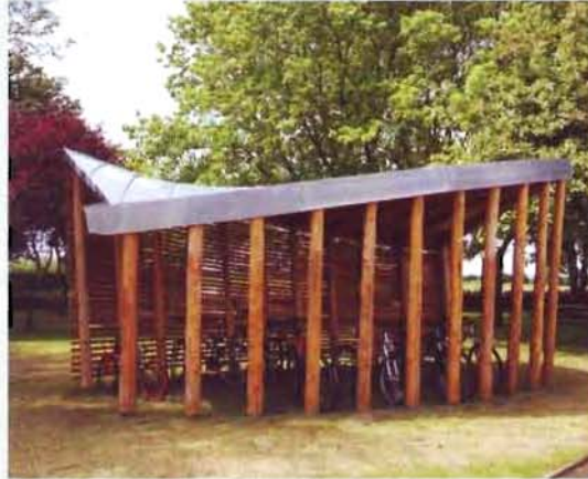
Locally grown larch timber was used for the shelter.
