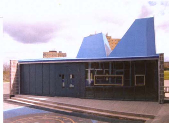
Left Two canted towers dominate the roof's profile Above The roof is clad with bright blue Sarnafil membrane Right Rooflights in the
