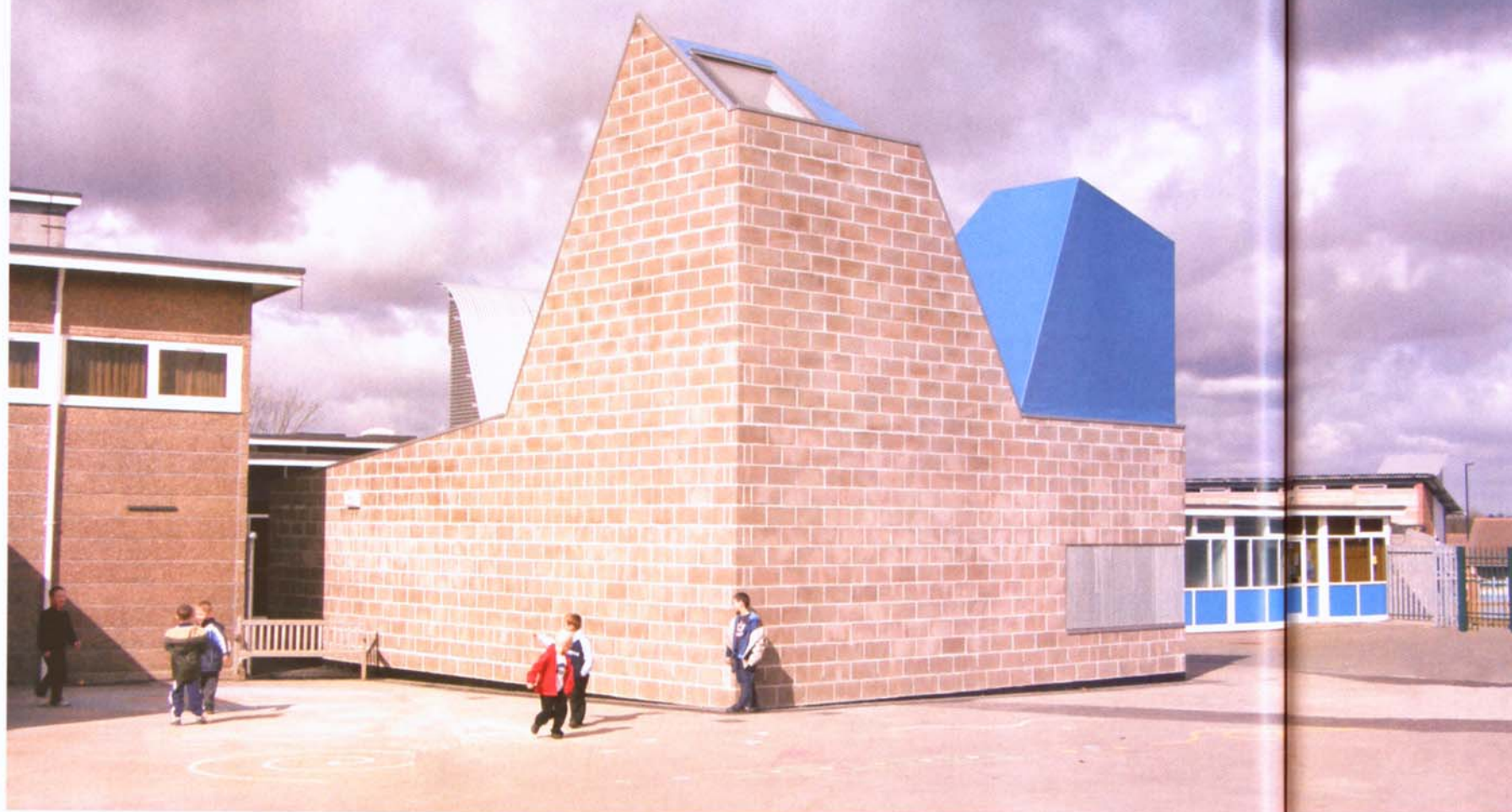
Left Two canted towers dominate the roof's profile Above The roof is clad with bright blue Sarnafil membrane Right Rooflights in the
